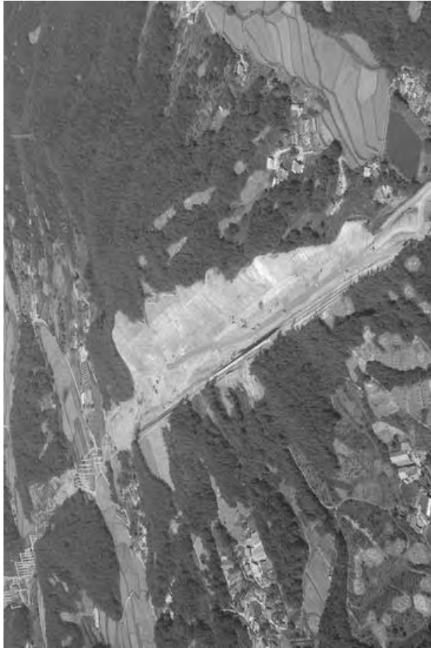
Road Construction Site
