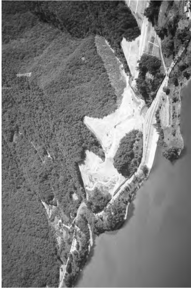
Road Construction Site
